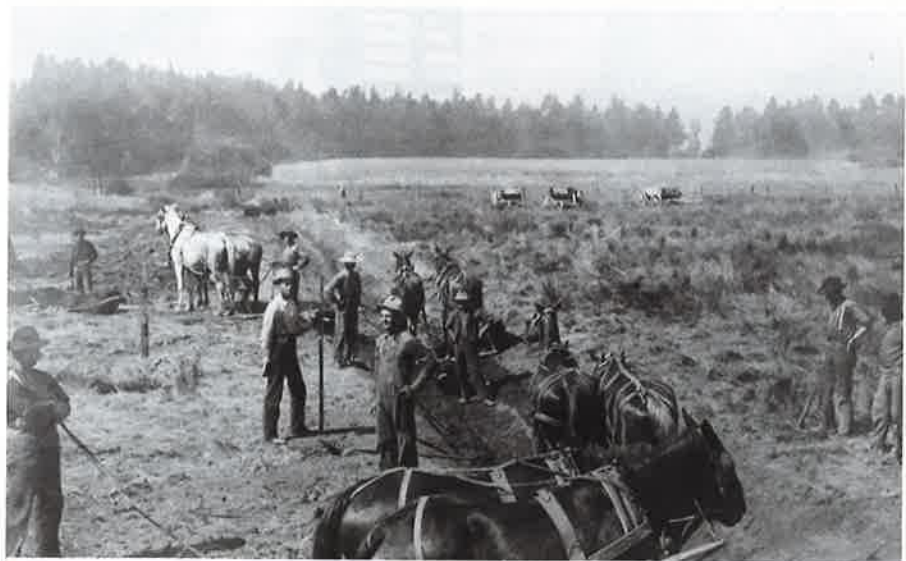
Figure 2: Diking of salt marshes in San Mateo, Alameda, and Marin Counties, CA, circa 1906-1910; courtesy of Alameda Mosquito Abatement District.
