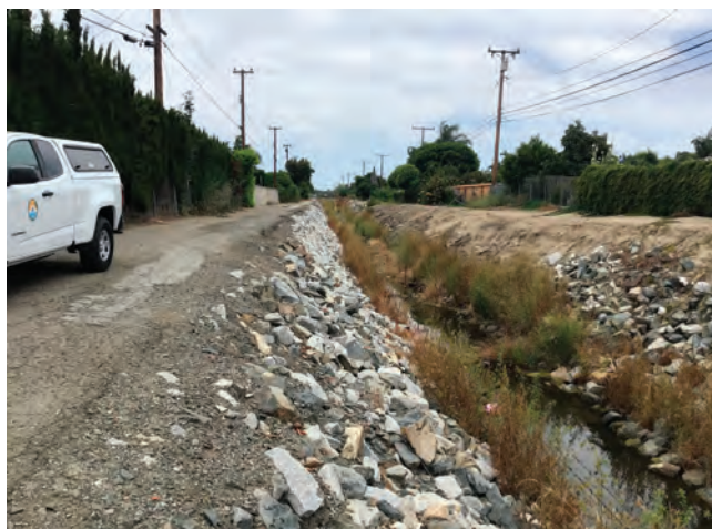
Figure 1.—OCMVCD identified this OC Public Works Flood Control channel as a significant mosquito source due to persistent water and unmaintained vegetation.
