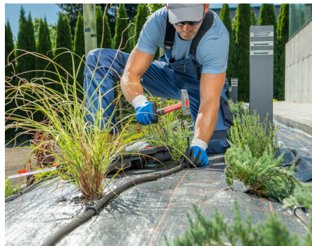
Landscaper installing a new drip irrigation system to decrease standing water
