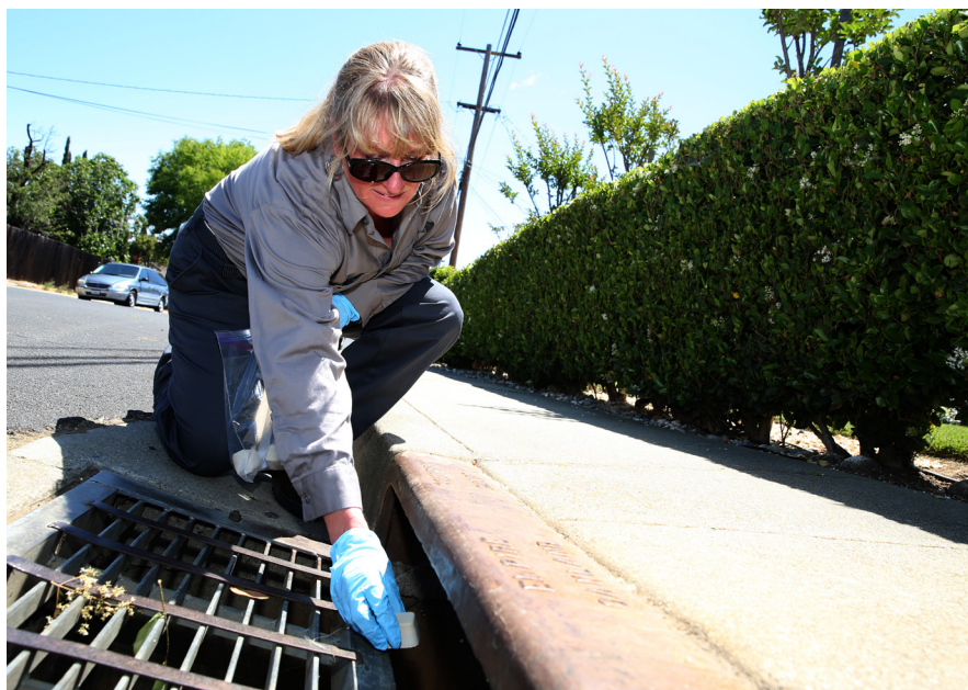
A vector control technician treats a stormwater catch basin with a larvicide tablet.
