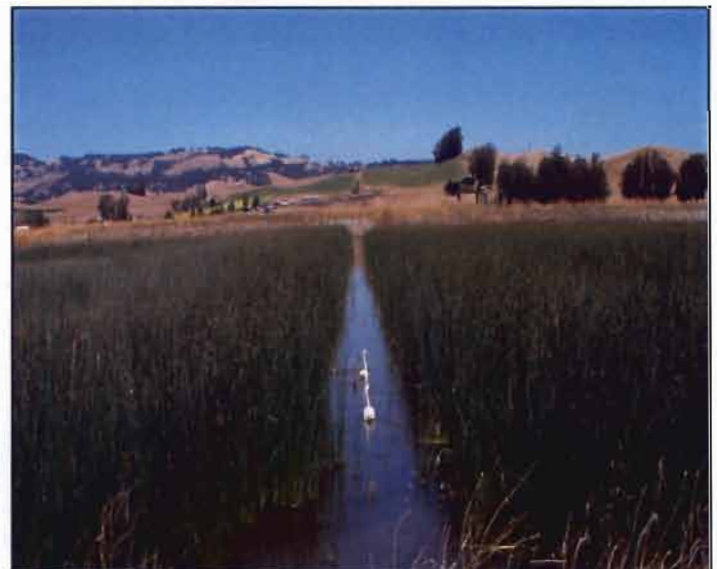
Figure 3. Petaluma waste water treatment facility pond covered with bulrush.
