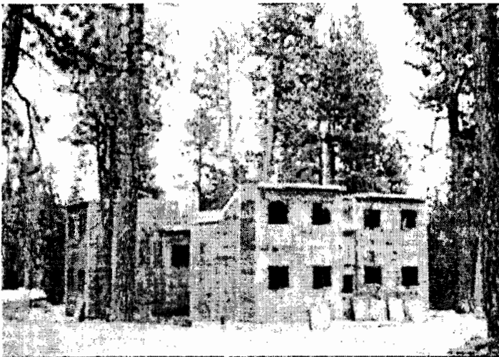
Figure 2. A barracks at a Forest Service facility, Mono County, California (Site #1). The site of several confirmed and suspect TBRF cases.
