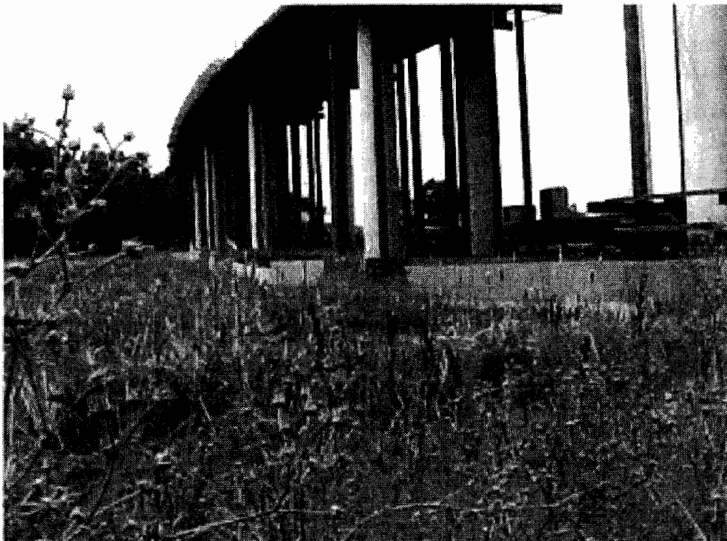
Figure 4. Snake exclusion fencing around construction site at Mills Field.
