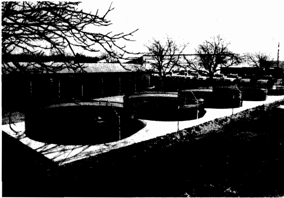
Figure 2.-The completed mosquitofish holding facility consisting of five circular tanks.
