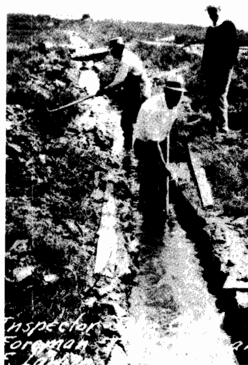
Figure 3.-Ditching the marsh, 1935.
