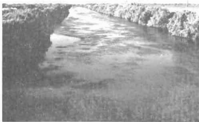
Figure 3.—Outfall drain at the lower end of Palo Verde Valley, collecting and carrying water from other drains. Drains of this type have good water flow at all times, full of mosquito fish and other predators, and no potential for mosquito breeding exists here.
