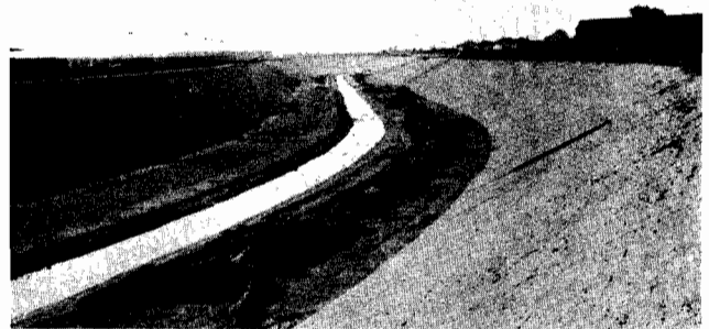
Figure 2.—Part of the East Fork of Coyote Creek adjacent to residential-industrial establishments, Los Angeles County, California, where the substrates from the channel were removed.
