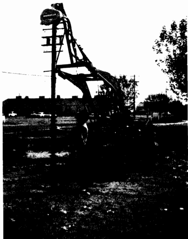
Fig. 1.—Drilling equipment used to obtain vertical drainage, showing hydraulic boring head and 6-inch auger with extensions.
